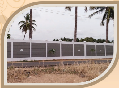
Compound wall provided for the Entire layout
