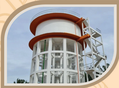
Ovre Head Water Tank
