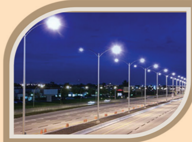
Electricity Lines with LED Lights
